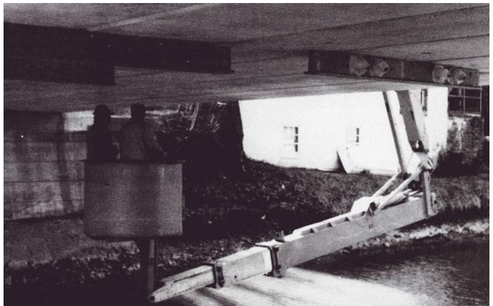
Installing beams with artificial nest sites.
